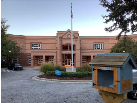
1). Northeast Elevation - Dec 19, 2019
