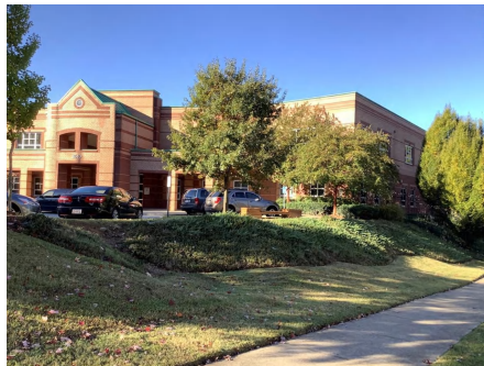
8). North Elevation - Dec 19, 2019
