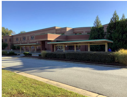
5). Southwest Elevation - Dec 19, 2019
