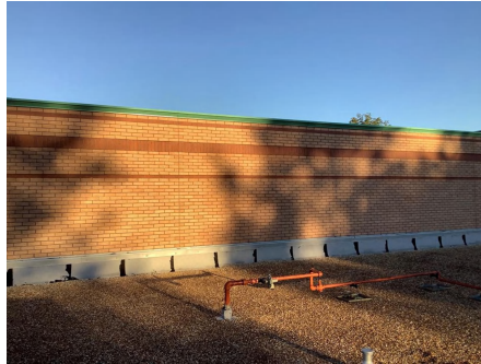
2). East Elevation - Dec 19, 2019
