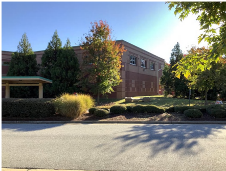
4). Southwest Elevation - Dec 19, 2019
